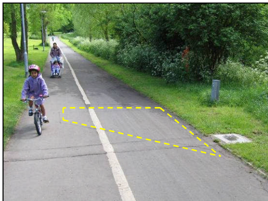
Inductive detection loops (highlighted) not covering full width of path
