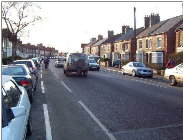
Removal of Road Centre Lines, Peterborough (note absence of buffer zone between parked cars and cycle lane: see A11 Cycle Lanes )
